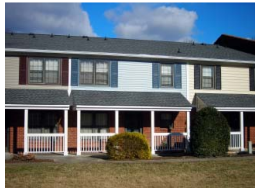
Glendare Apartments - after
